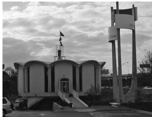
Formerly a Trust Company Bank branch designed by Henri Jova and built in 1962, piebar is a sleek rehabilitation of modern architecture in Atlanta.
