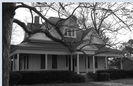
E.M. ROGERS HOUSE , Adel, c. 1907. Purchased in 1913 by E.M. Rogers for his bride, the one-story Queen Anne cottage features 14' ceilings, heart pine floors and a steeply pitched hipped roof. The 2,000-sq.-ft. house also contains 6 fireplaces, 7 rooms and 2 full baths. The surrounding 1/2-acre property includes 3 outbuildings. $149,500. Contact Frank White at 404-885-7807.
